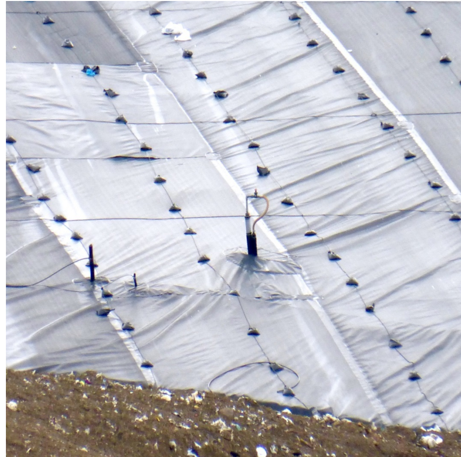
Final Cap with Wells
